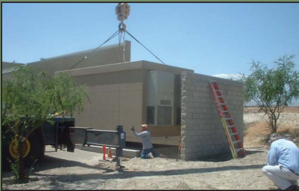
Pictured from top: One Wilshire Building (Los Angeles, CA), Installation of CalREN Palm Desert backbone node (Palm Desert, CA)
